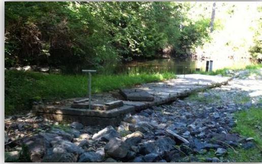
The water is transported approximately 2.5 kms down the hill and under the inlet to the Bay Street water treatment building and pump station. The supply line is reported to consist of 520 m of 350 mm diameter pipe connected to 1,300 m of 250 mm diameter pipe which connects to 690 m of 300 mm diameter High Density Polyethylene (HDPE) submarine pipeline.
