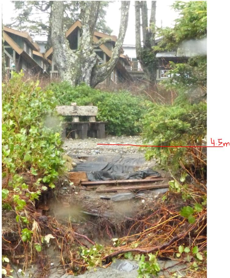
Figure 48: Erosion of an engineered shoreline at Terrace Beach. Estimated observed elevation is 4.5 m, modelled runup elevation is 5.5 m. Photo credit: John Towgood.
