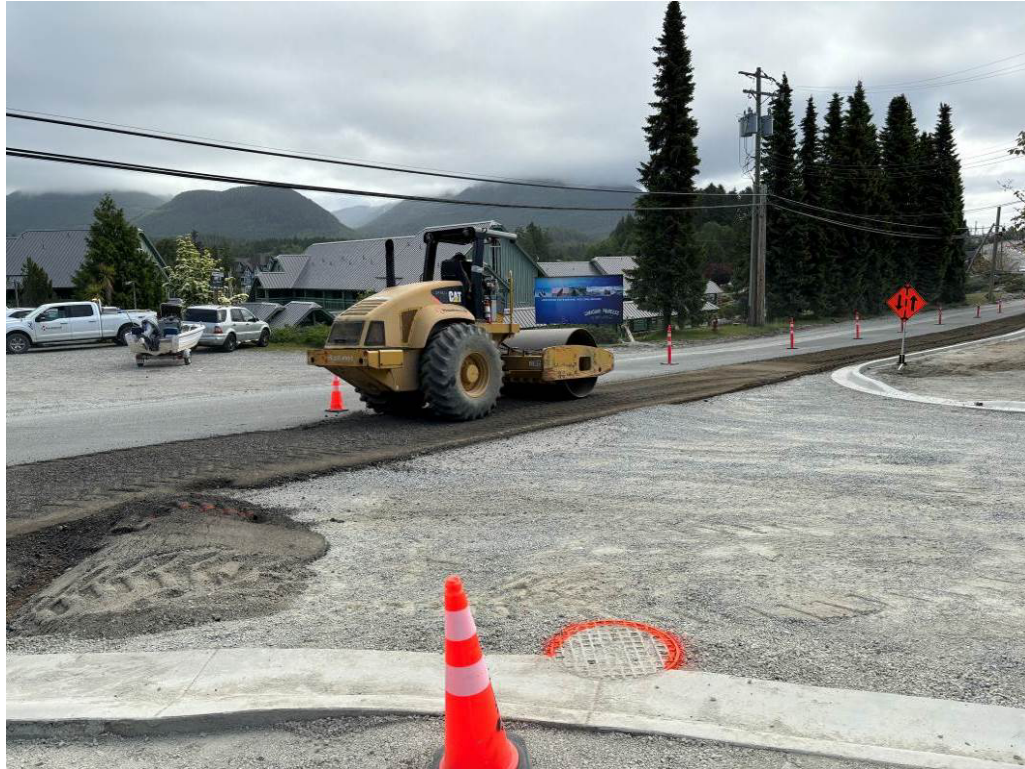
Photo #3 – Roadway Compaction Ongoing
