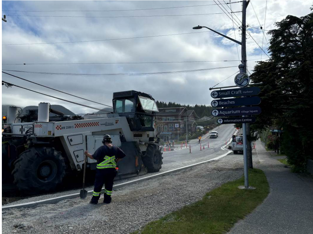
Photo #1 – Roadway Pulverizing Completed
