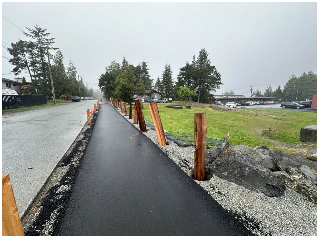
Photo #2 – Split Rail Fencing Post Installation Ongoing
