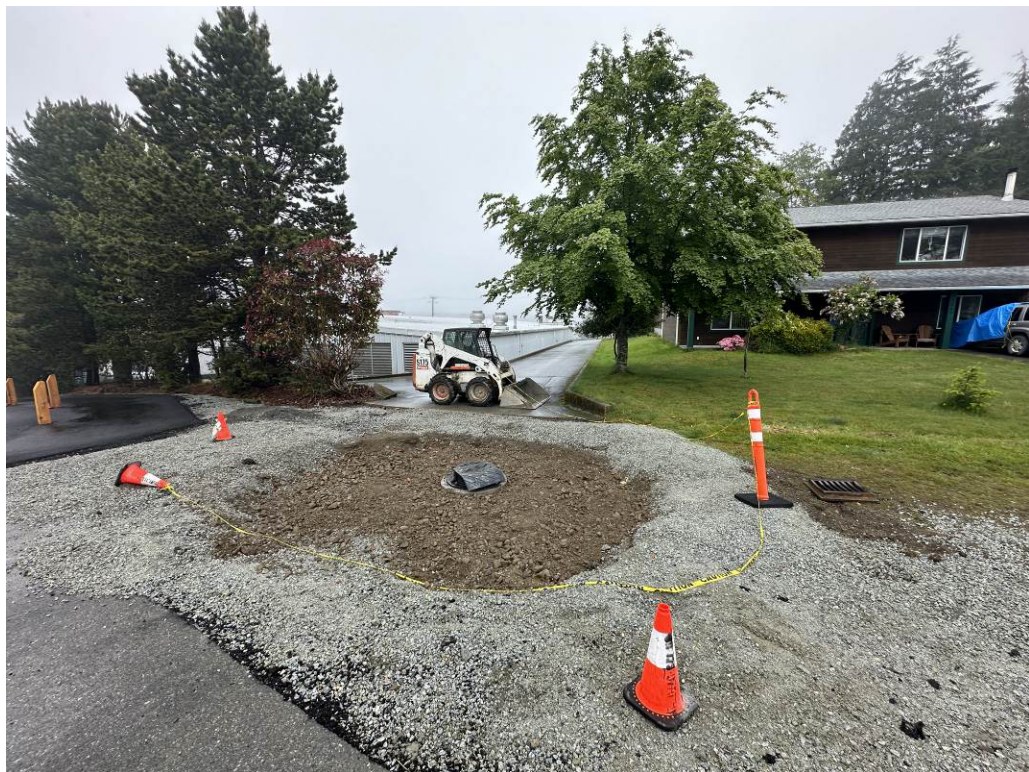
Photo #6 – Catch Basin Replacement at Asphalt Lane (Back of CO-OP)
