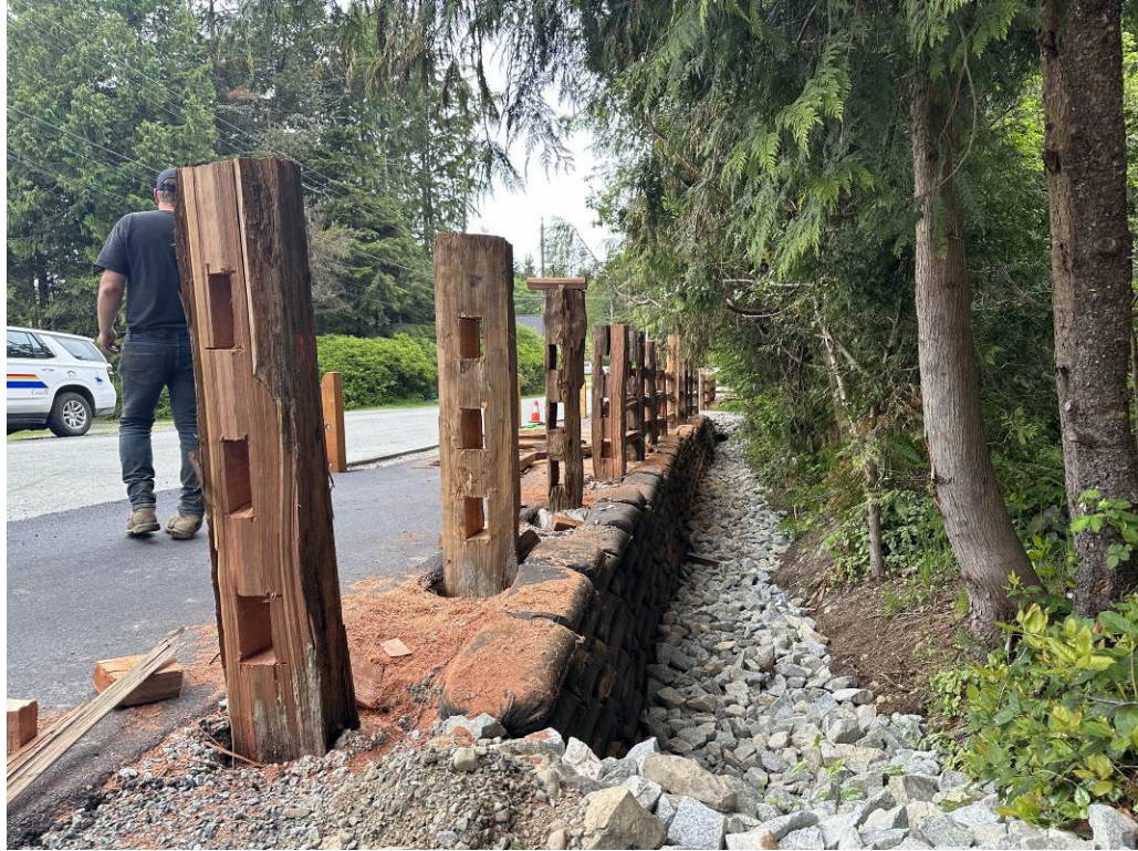
Photo #5 – Culvert and Ditch Armoring
