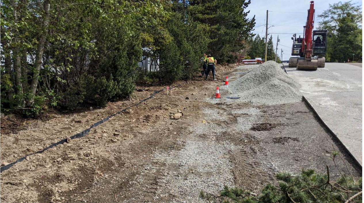
Photo #3 – Root Guard Installation Completed (Sta. 5+340 to 5+390)
