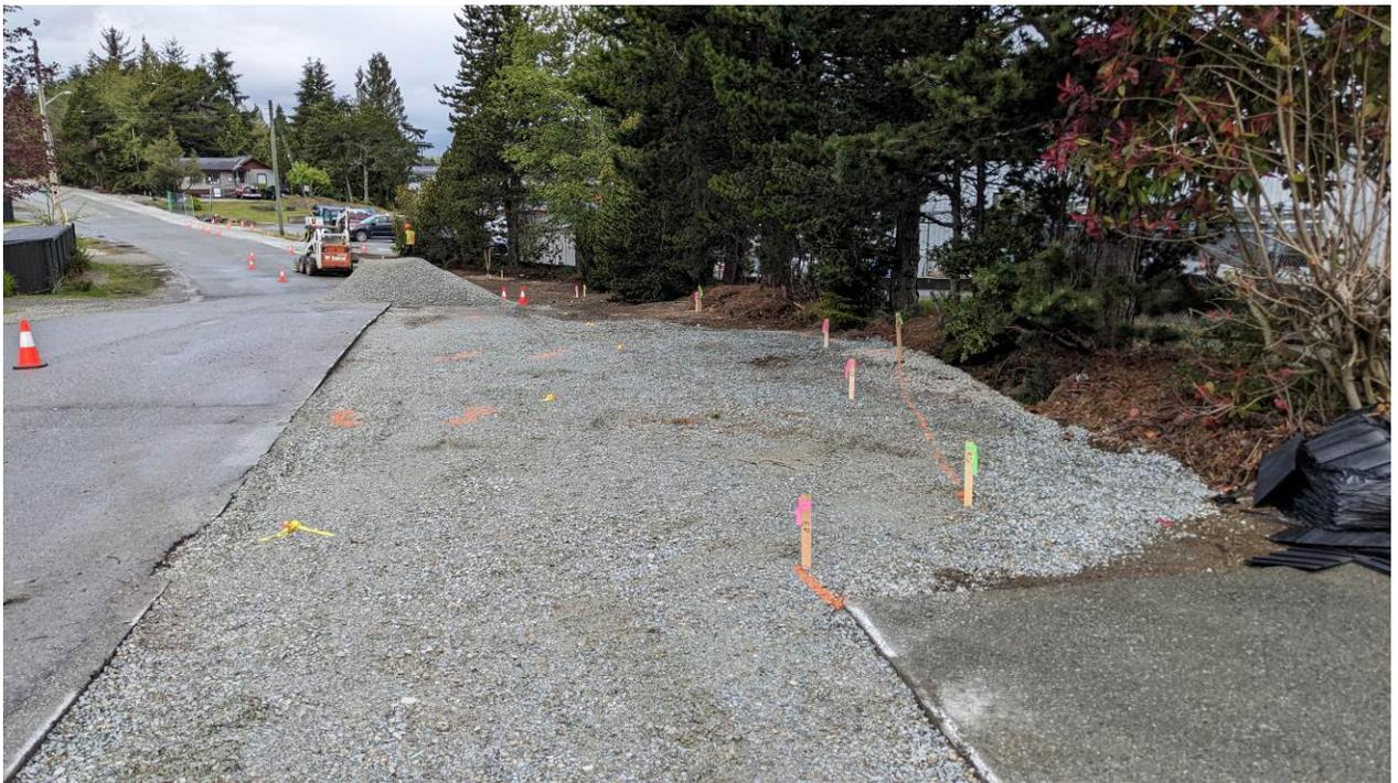
Photo #2 – Larch Road Pathway – Roadway Widening in Progress (5+400)
