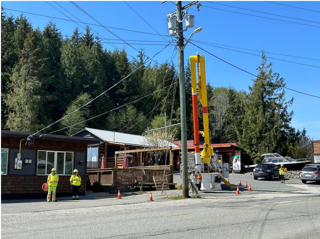
Photo #8 – Sidewalk Guy Installed on New Anchor
