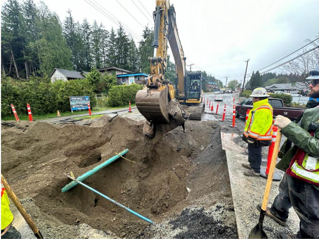
Photo #5 – Removed Existing Pipe (CSP)
