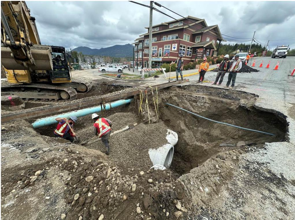
Photo #2 – Concrete Pipe Installed from DMH #11 towards DMH #6
