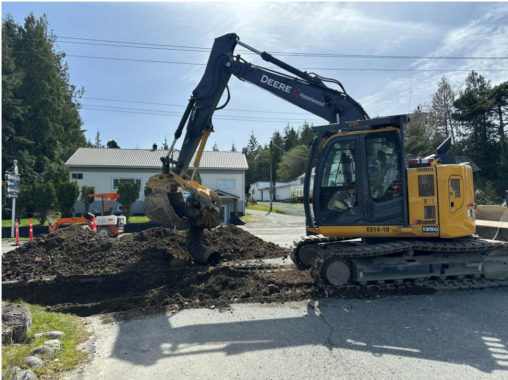
Photo #6 – Removed Existing Pipe (CSP) along Peninsula Road
