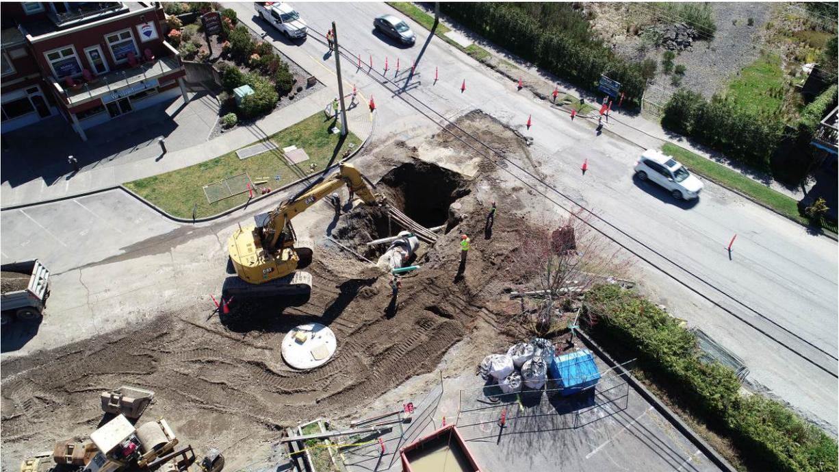
Photo #6 – DMH #11 & Concrete Pipe Installation Near Lyche Road
