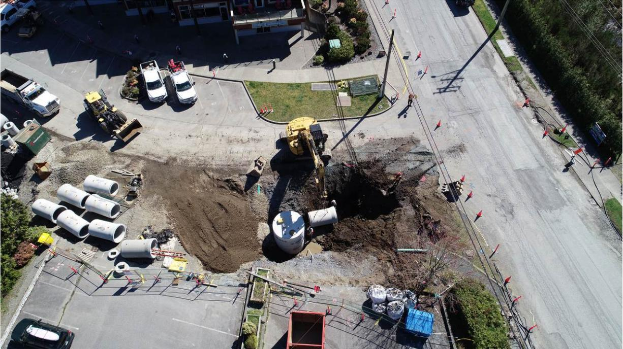
Photo #5 – DMH #11 & Concrete Pipe Installation Near Lyche Road
