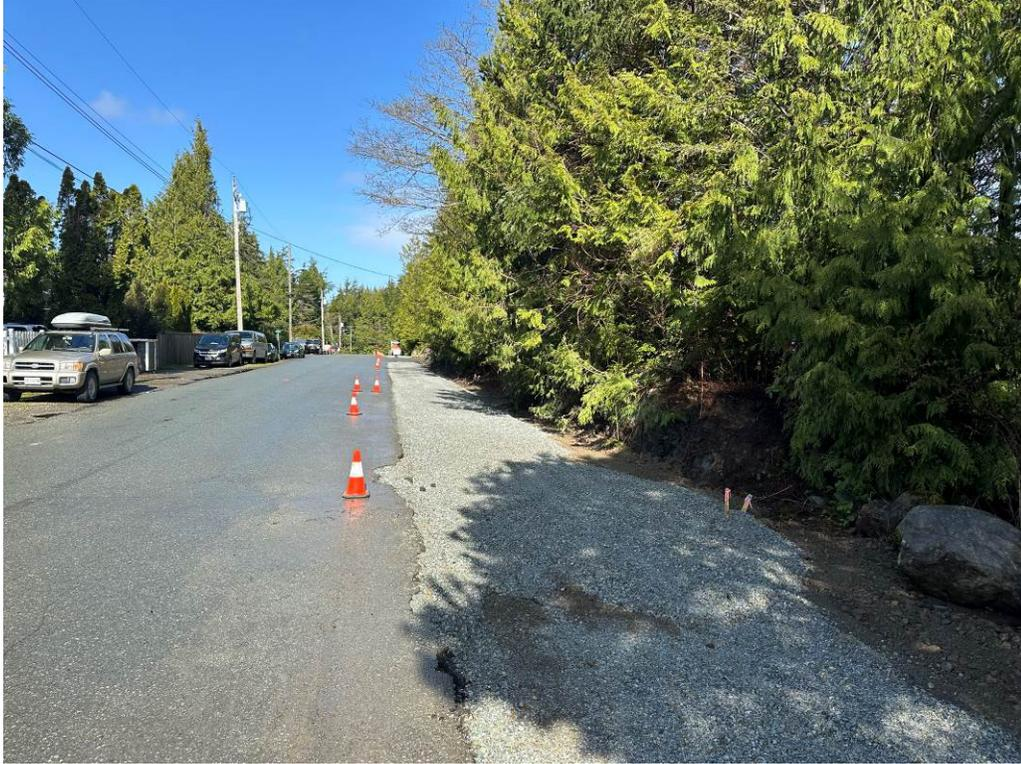
Photo #1 – Larch Road Pathway – Roadway Widening in Progress (5+200)
