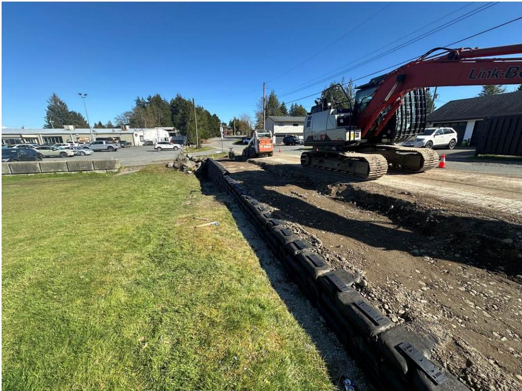
Photo #4 – MSE-Flex Wall Construction Ongoing (Sta. 5+300)
