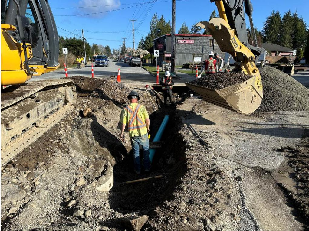
Photo #1 – New Catch Basins at Bay Street Connected to New System
