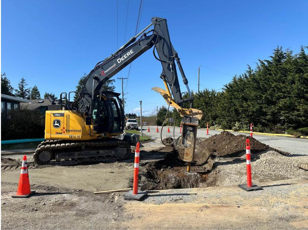
Photo #3 – Rock Removal Completed for Bay Street Drainage Improvements
