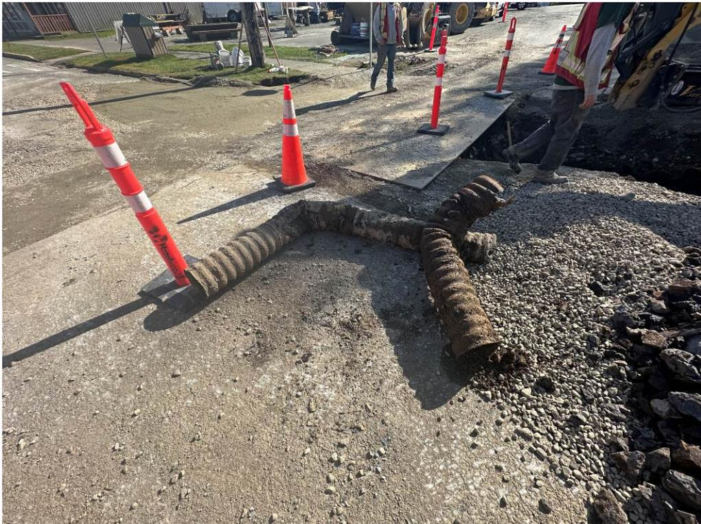
Photo #2 – Existing Pipe at Bay Street Removed
