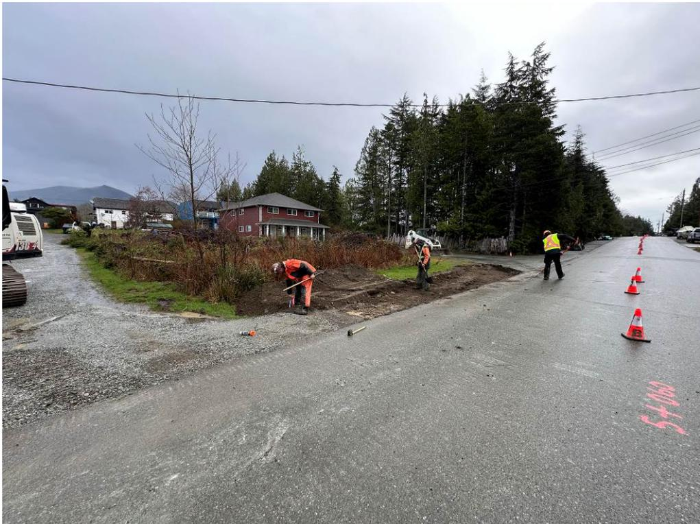
Photo #4 – Larch Road Pathway – Roadway Widening in Progress (5+060)
