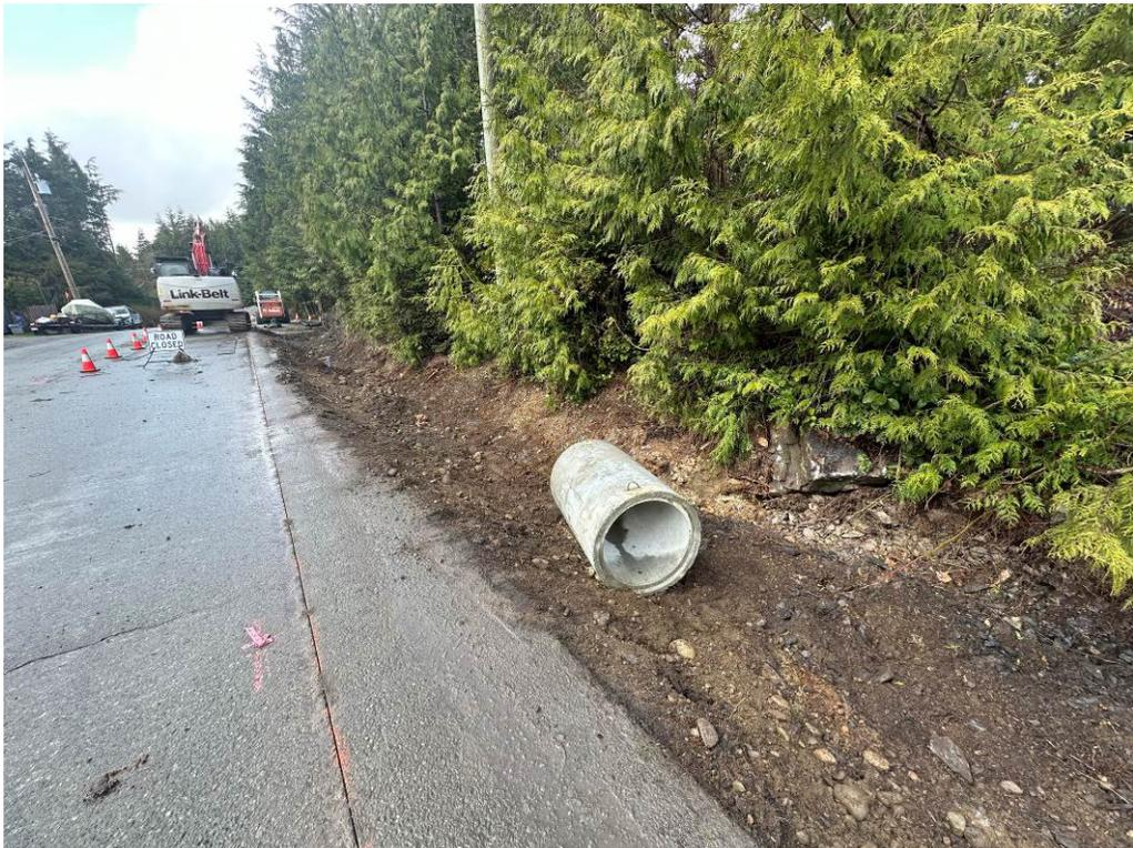
Photo #2 – Prep for Bio-Swale / Storm Pipe Installation (Sta. 5+170)
