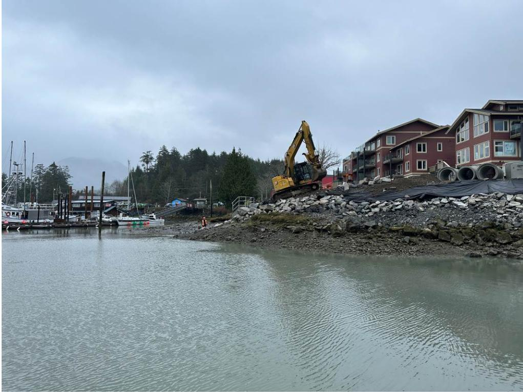
Photo #5 – Final Rip Rap Placement at Outfall completed during low tide (with environmental monitor onsite)
