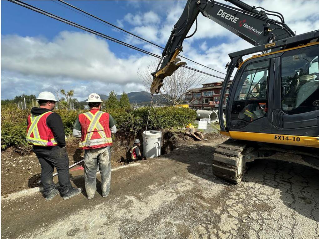
**Photo #1 – New Catch Basins Installed**
