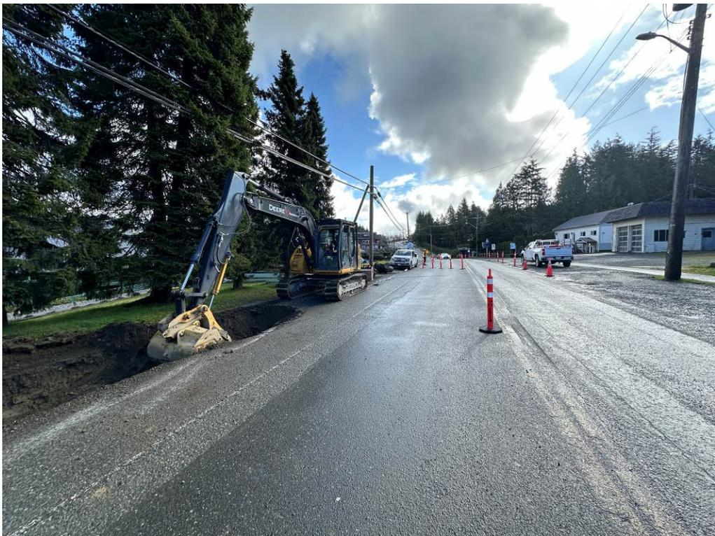
**Photo #2 – Old Storm Pipe (CSP) Removed (Along North Side of Road)**
