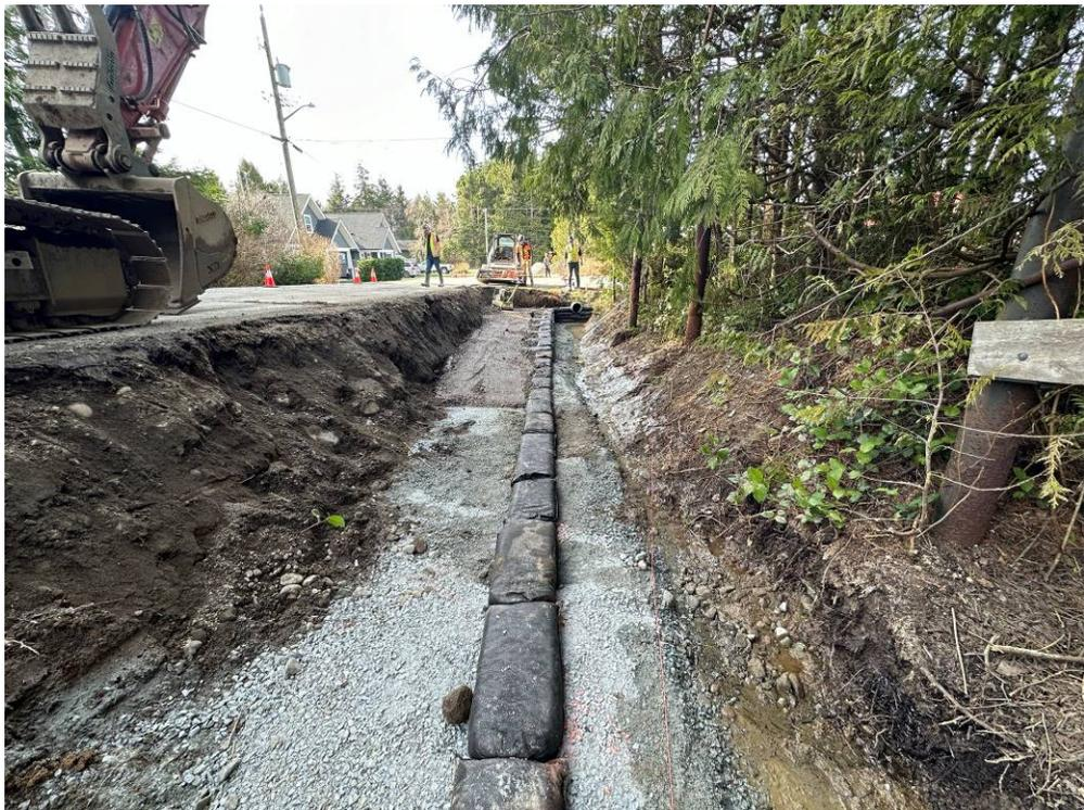
Photo #2 – Installation of MSE bags and backfill
