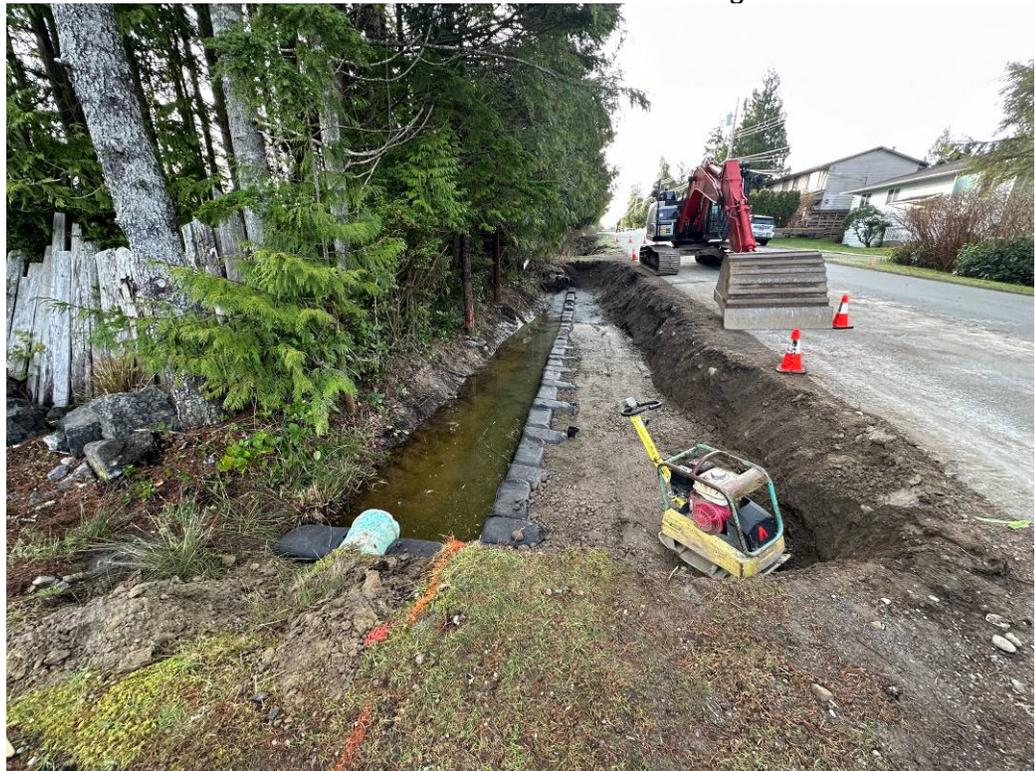
Photo #4 – MSE Wall Backfill and Compaction (STA 0+090)
