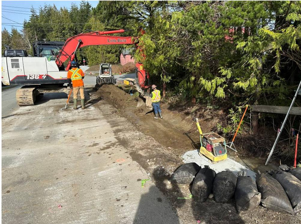
Photo #1 – Excavation and base prep for MSE Wall (STA 0+090)
