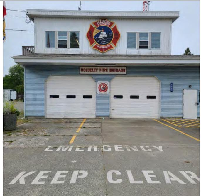
Ucluelet Fire Hall front elevation view from Peninsula Rd. Main Fire Hall concrete apron marked for emergency use only. Concrete apron shows significant signs of wear and degradation. Ucluelet Fire Brigade branding is being updated. Street frontage shows building past life cycle.
