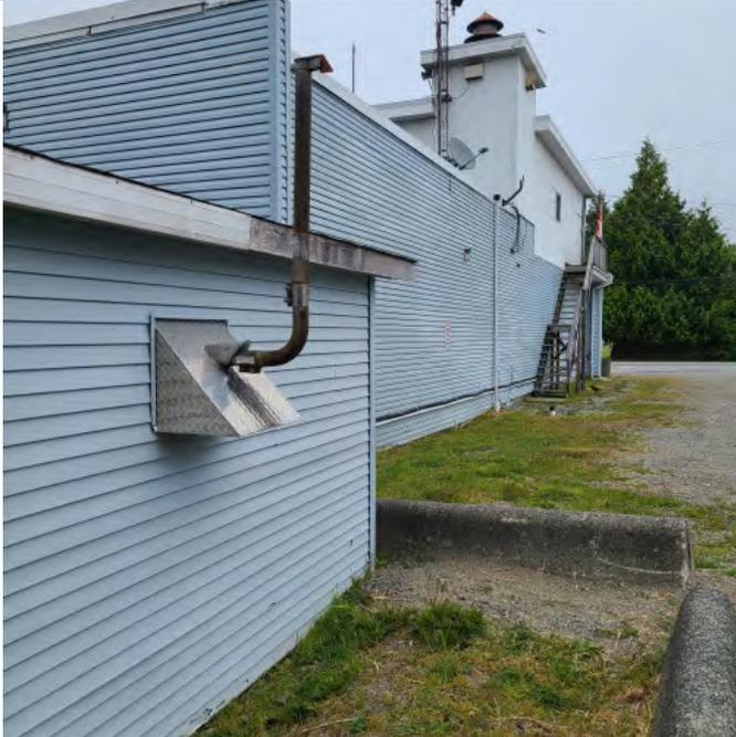
The photo above shows significant organic growth along the building facades. The buildings show outdated architectural and building envelope details. Fascias and flashings are deteriorating.
