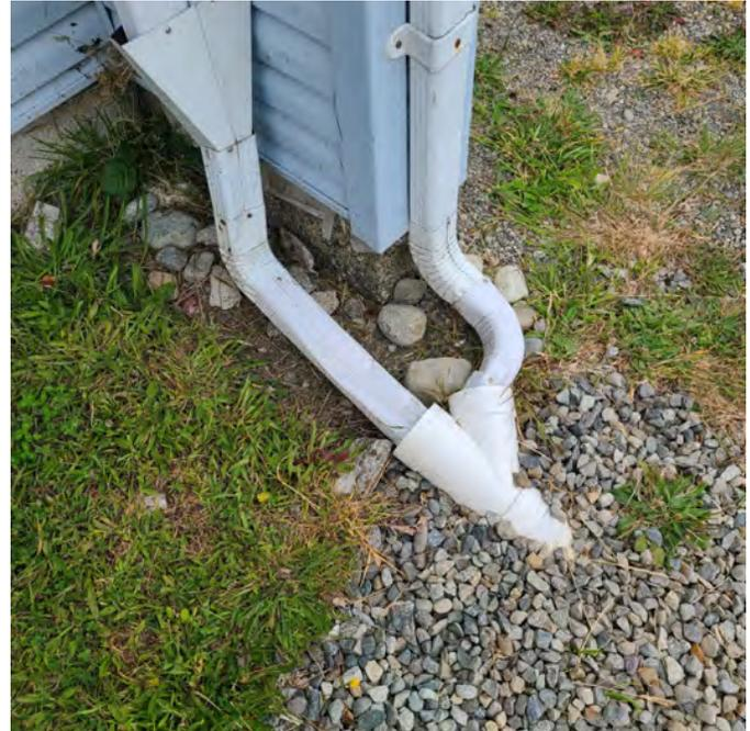
The photo above shows that while SOME perimeter storm drainage is installed, it has not been installed properly and appears to not be installed at the required depth for frost protection. This installation would fail a current building inspection.
