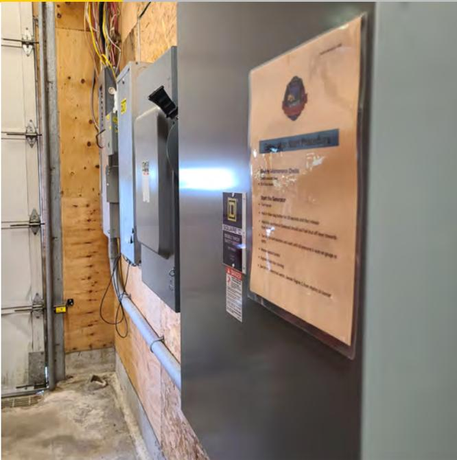
See previous photo notes. Additionally, daylight can be seen along the edges of the overhead door resulting in significant energy loss.
