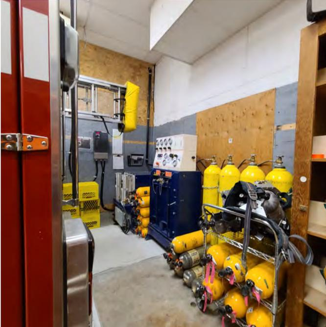
The photo above shows the SCBA and compressor station. The fill station is positioned at the rear of the apparatus bay and has potential for exhaust contamination. Functionality and movement in this area is very limited due to the small space.
