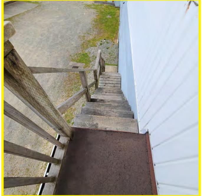
The photo above shows a view from the exterior exit stair landing to the ground. The landing surface is deteriorating and narrow. The hand rail is not of an acceptable design. NOT TO CODE/ unsafe for use.
