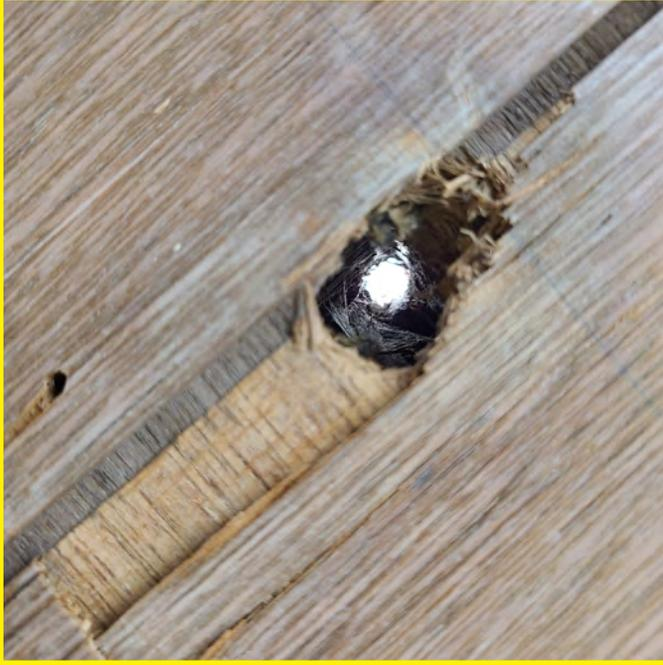
The photo above shows a hole through the complete building envelope. Daylight can be seen from the interior. The building wall assembly does not appear to be acceptable.
