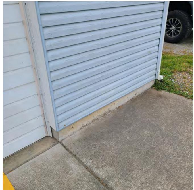
The photo above shows OH door weather protection detail issues. Water may enter the apparatus bays during major rainfall or significant wind driven rainfall events with inadequate sloping and lack of slab drainage.
