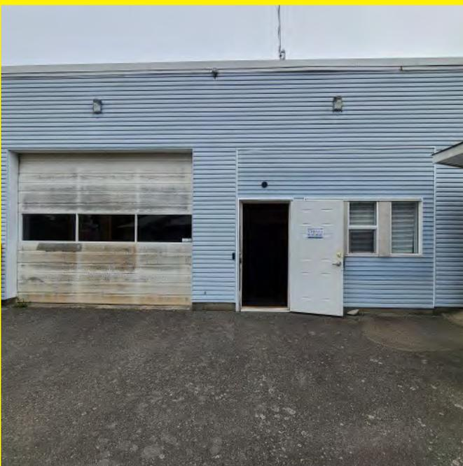
The photo above shows the overall facade deterioration and inadequate site lighting. Lighting should be upgraded to LED for energy efficiency. Windows and doors should be replaced for improved energy efficiency. No door panic hardware for exiting.
