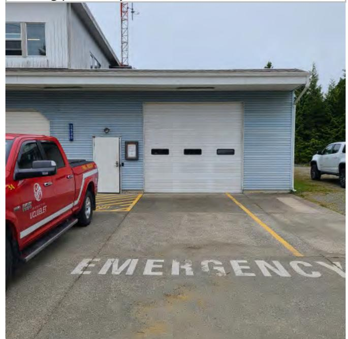
Added apparatus bay. Overhead doors are smaller than industry standard. Needs 12'Wx14'H min. size.
