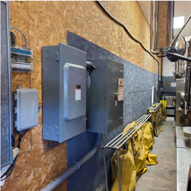
The photo above further shows that movement is limited around all sides of the trucks in the fire hall. Electrical equipment needs relocation to a proper electrical room.
