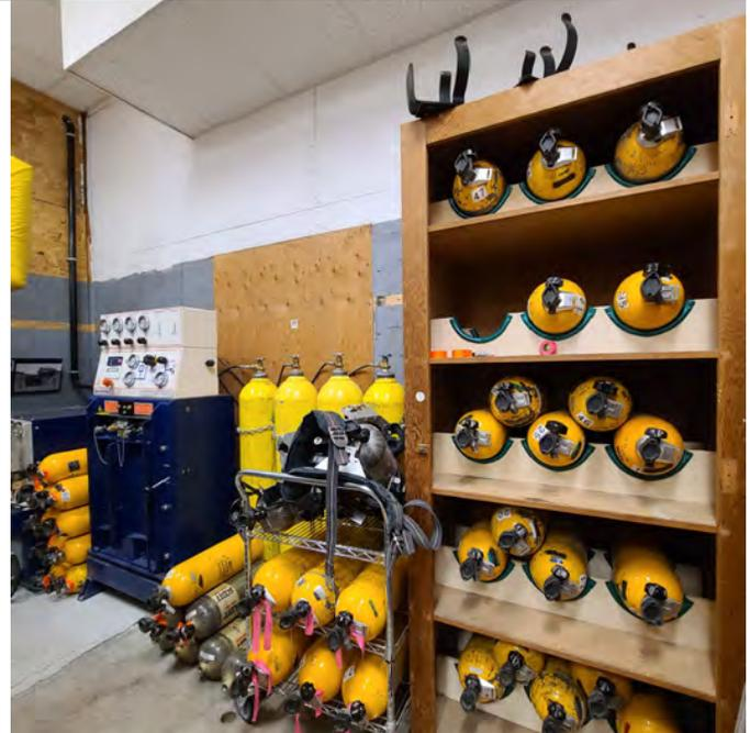
The photo above further highlights the issues noted in the photo to the left. SCBA and compressors required a dedicated 'clean room' for proper separation from apparatus bays and intake of fresh air. Clean work area is needed for storage and maintenance of equipment.
