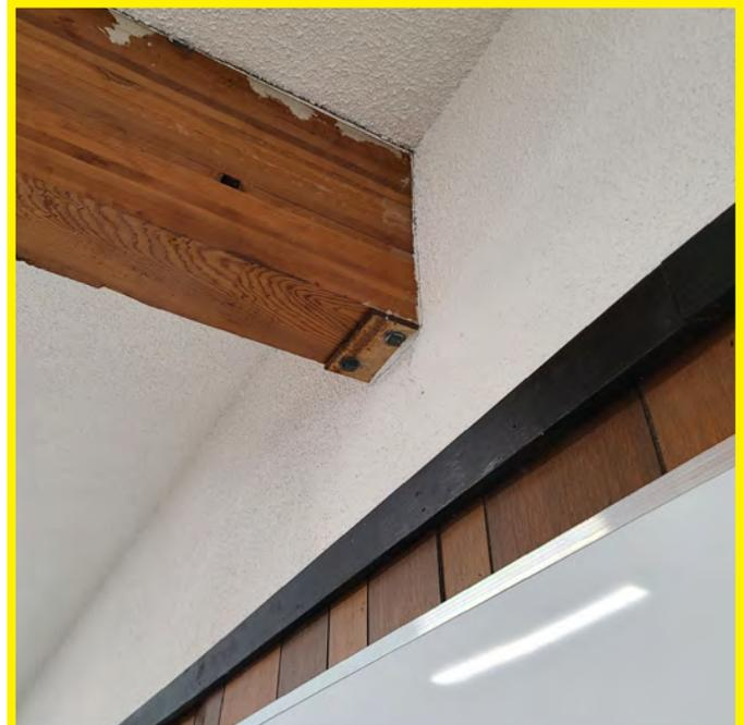
The photo above shows the glulam beam support at the front exterior wall. The beam is fastened to a metal bracket. The integrity and adequacy of this connection cannot be confirmed. It does not appear seismically sound.
