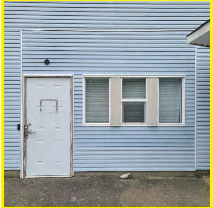
Photo above shows patchwork to building envelope and inadequate window and door details. It is assumed that the building envelope has completely failed and no longer keeps out water from the wall assembly. Windows are old and past product life cycle.
