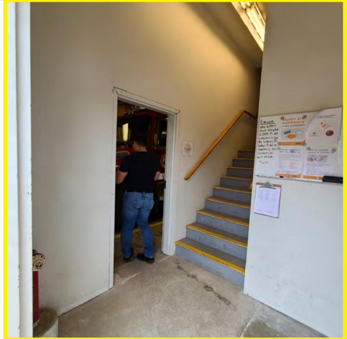
The photo above shows the existing condition of the bare concrete flooring. No concrete sealer appears present or has worn away. The areas of addition are seen. The **fire rating** of this exit stairwell cannot be confirmed adequate.
