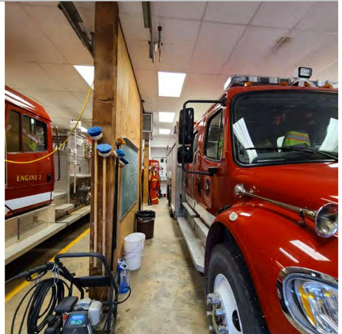
The photo above shows the space between the two original apparatus bays. Movement is limited and the lack of storage space for washing equipment creates tripping hazards. It is also assumed that this dividing wall is load bearing but has no fire ratings.
