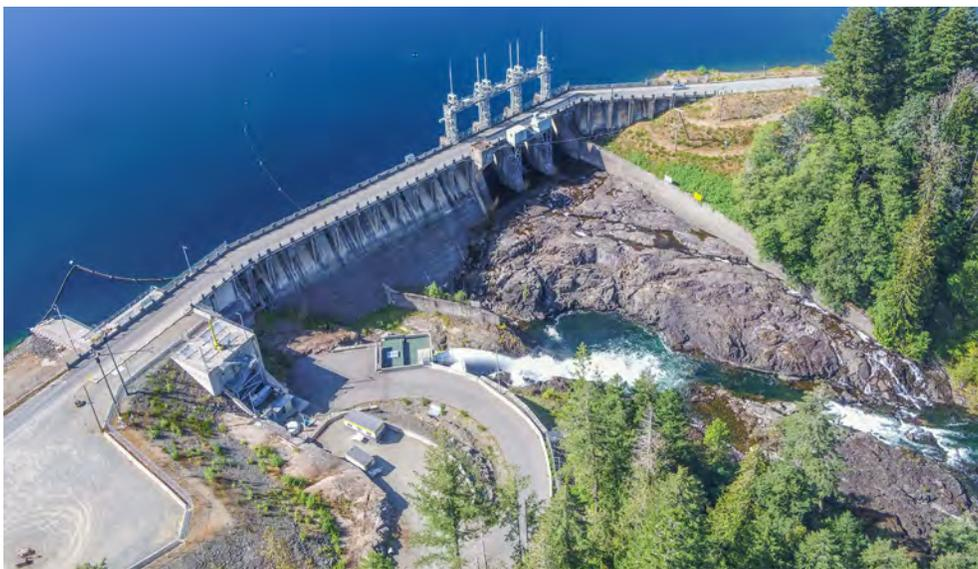
Site work has begun to prepare the area around the John Hart Dam in Campbell River for the upcoming John Hart Dam Seismic Upgrade Project. The Project includes seismic upgrades to strengthen the dam so it can withstand a severe earthquake. For more information on this project, as well as the Ladore and Strathcona projects, visit [majorprojects.ca](https://majorprojects.ca)
