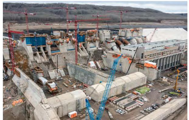
This aerial view shows Site C's spillways, penstocks, powerhouse and operations building for BC Hydro's third dam along the Peace River.
